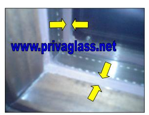
This kind of installation is ideal if your window/door frame is identical or similar to the one shown in the aside picture (double window pane with frame well along the window frame perimeter). Integrated installation means that LCD panel borders disappear into the perimetral window frame well and get sealed along with the window pane once the whole glass is inserted into the door/window frame.
